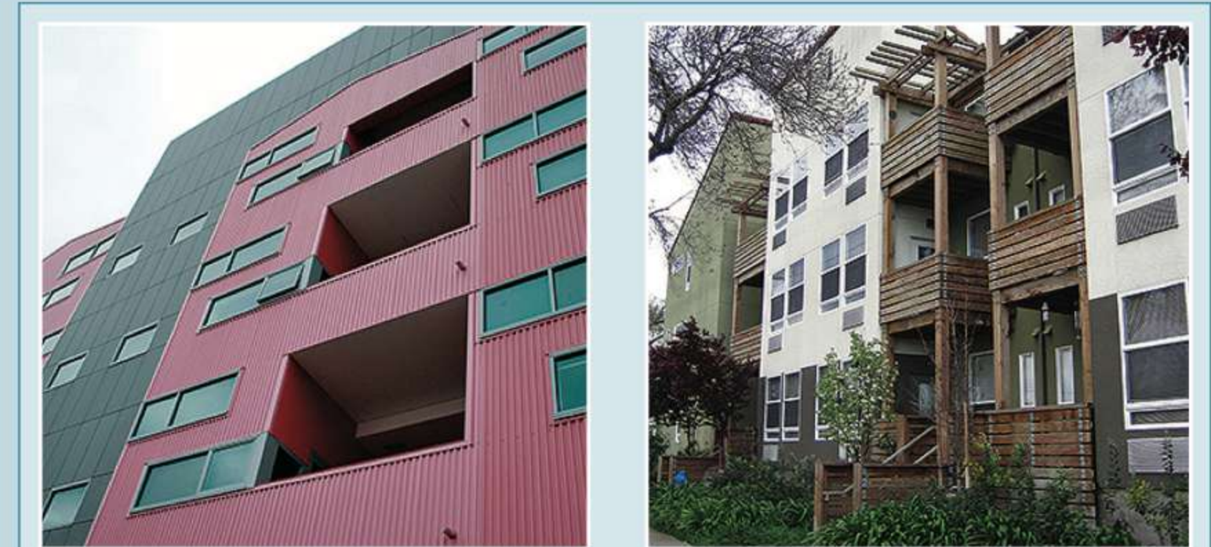
Figure 7: Building articulation variation in materials, colours and windows.
